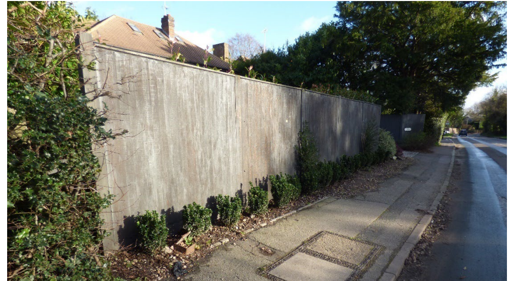
Figure 60: The removal of planting has had a suburbanising impact on some parts of the Conservation Area. In time the new planting will obscure the fence.
