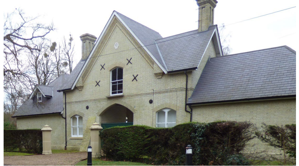
Figure 27: Castle Hill Stables features highly ornate brick and terracotta decoration on its gable and as part of its string course.
